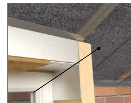
Abutment bracket is fixed to the infill timbers, angled panel bracket fixes to the wall.
